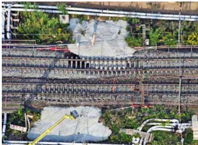
Concrete has been backfilled into the collapsed Rastatt rail tunnel
